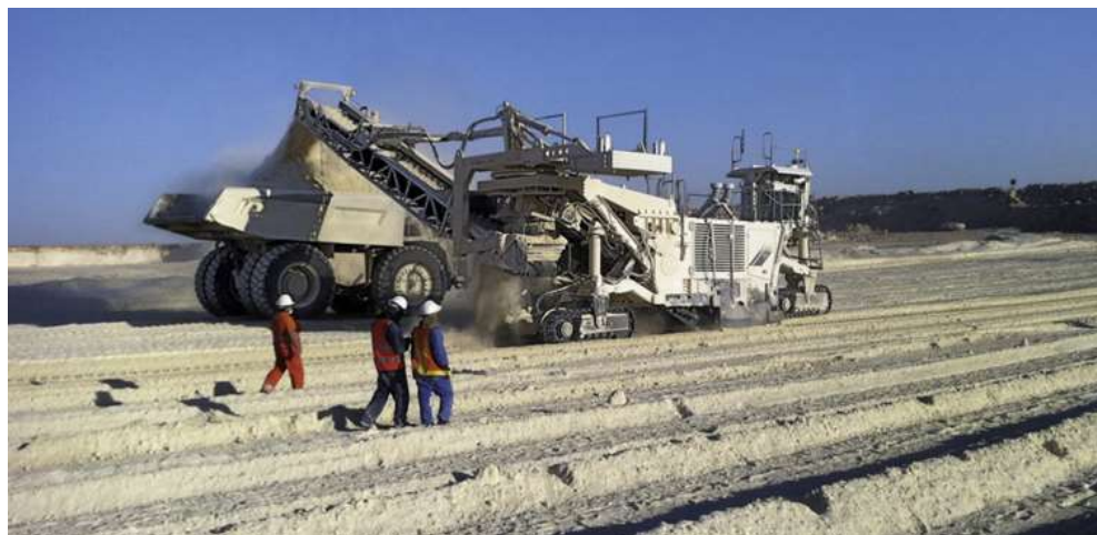
Fig 3 - Example Surface Miner – Limestone row cutting
