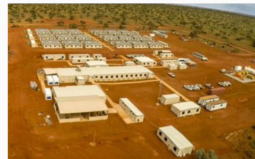
Image: Typical Site Accommodation Village
