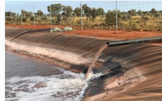
Image: Typical HDPE lined Water Pond
