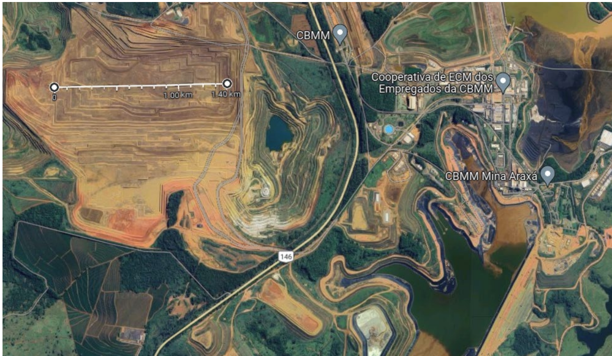
CBMM MINE AND PRODUCTION FACILITIES 1
