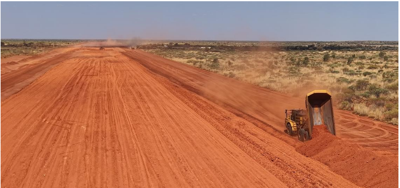
Figure 3: Construction of airstrip in progress
