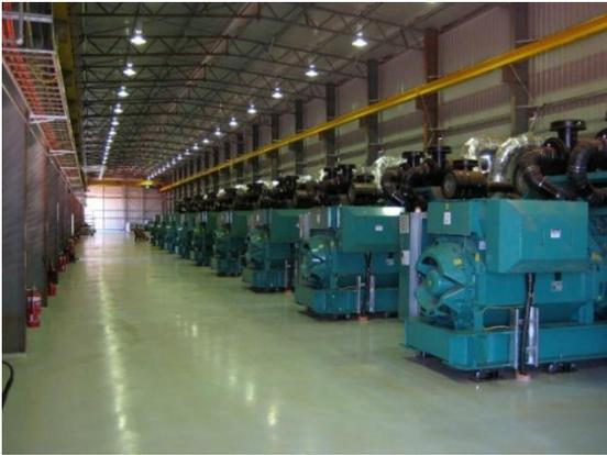
**Image:** Typical LNG-fuelled Engine Shed Layout
