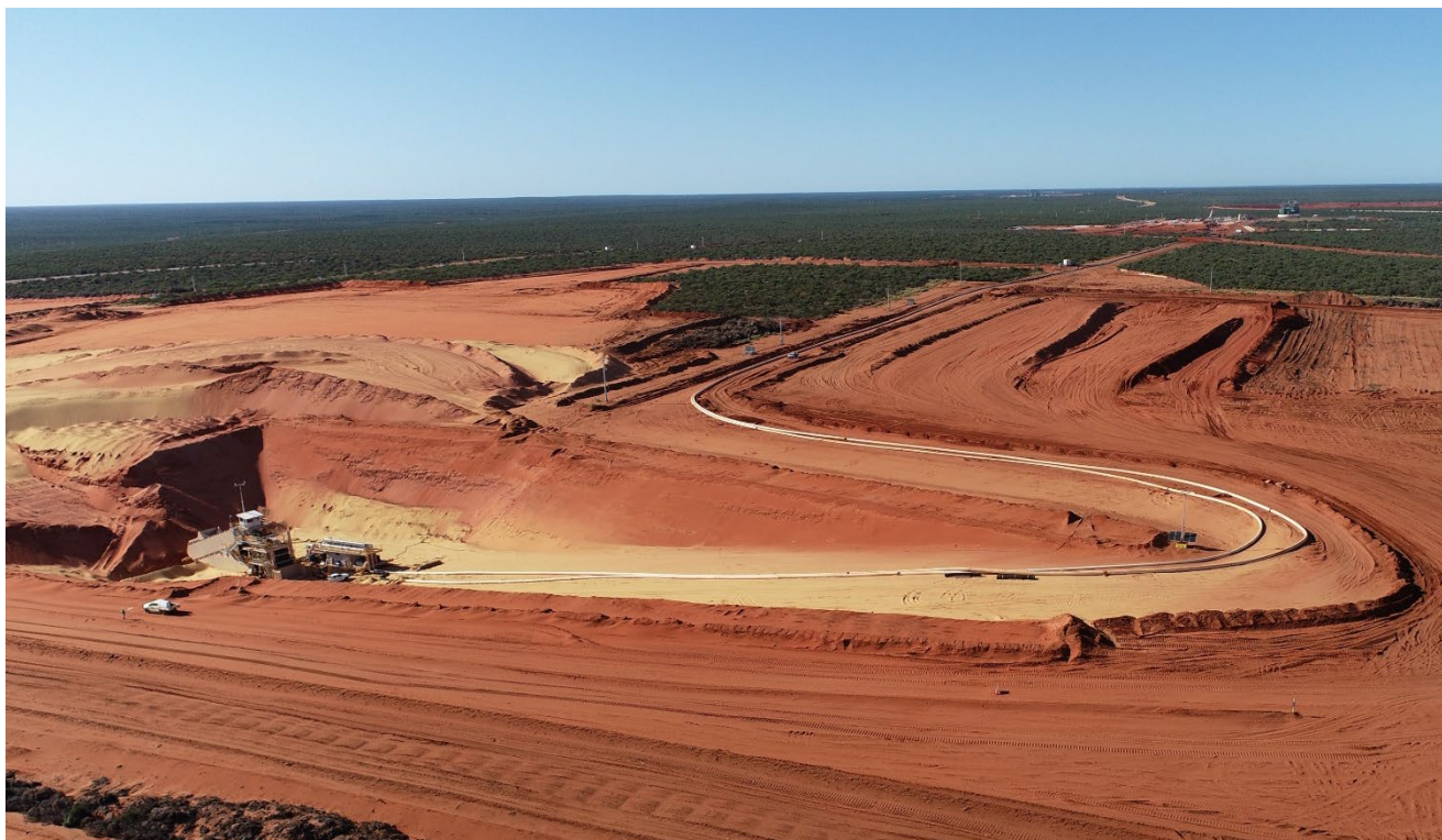
Figure 3 Pre-production development of Coburn's open pit mine is complete with all Dozer Mining Units connected
