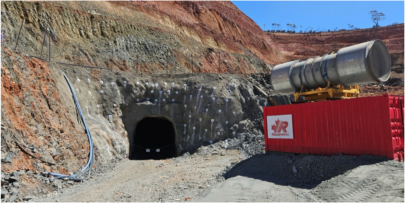
Figure 4 - Original Scotia North portal now rehabilitated.
