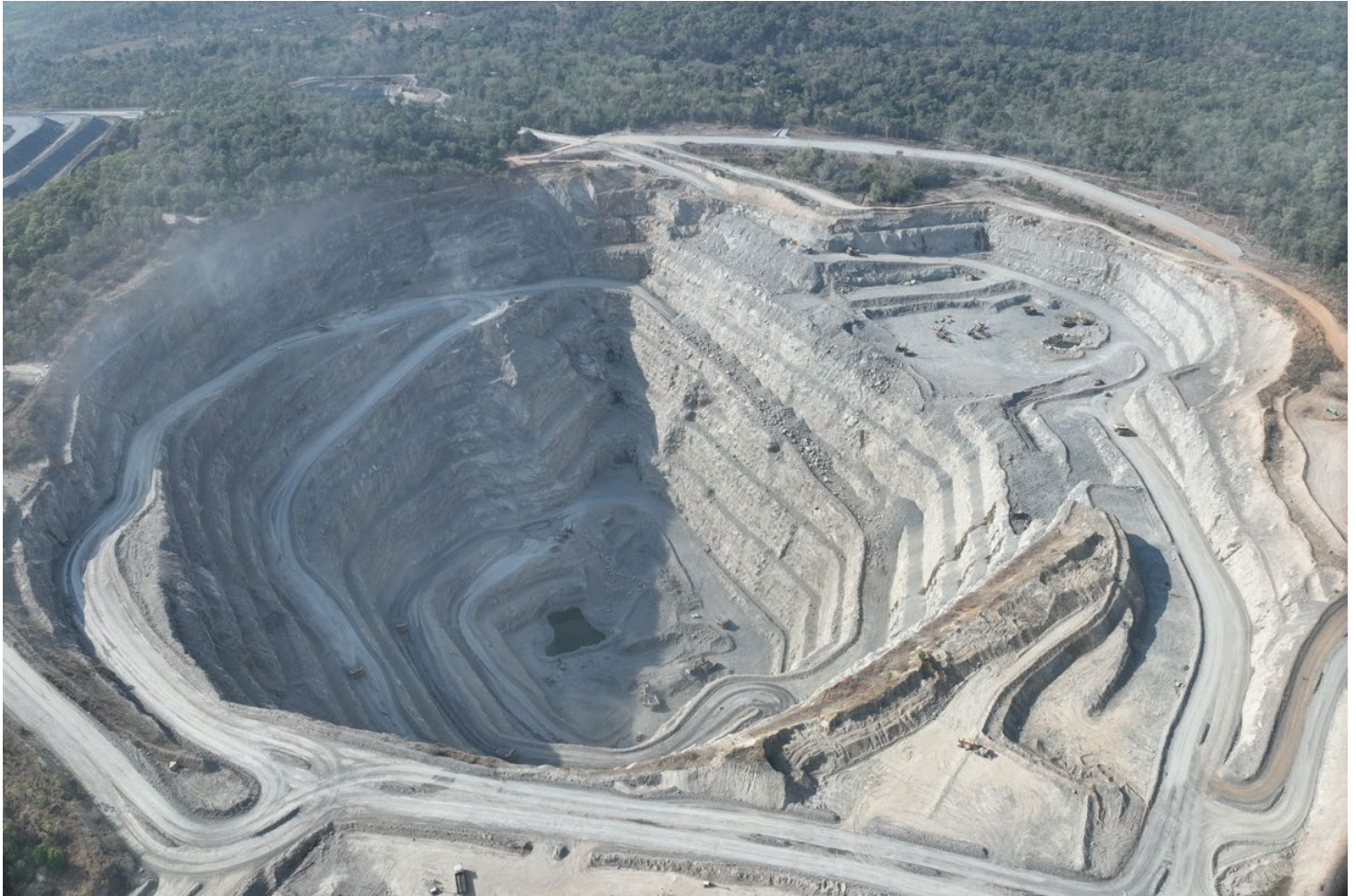
Figure 1 | Okvau Open Pit – April 2026
