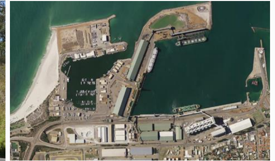
Image: Ariel View of Geraldton Port Infrastructure
