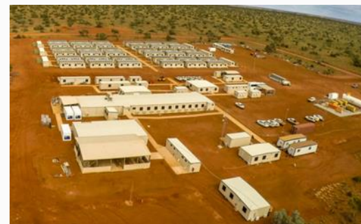
Image: Typical Site Accommodation Village
