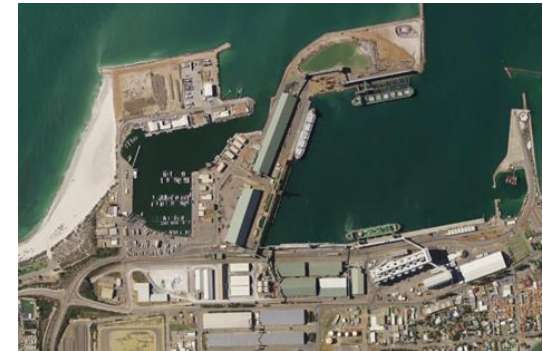
Image: Ariel View of Geraldton Port Infrastructure
