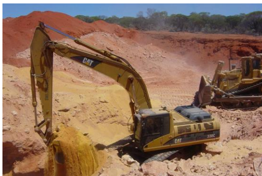
Image: Coburn Test Pit highlighting dry free flowing yellow sand with very low slime content, minimal loamy red sand and no calcrete
