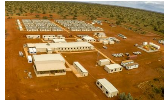
Image: Typical Site Accommodation Village
