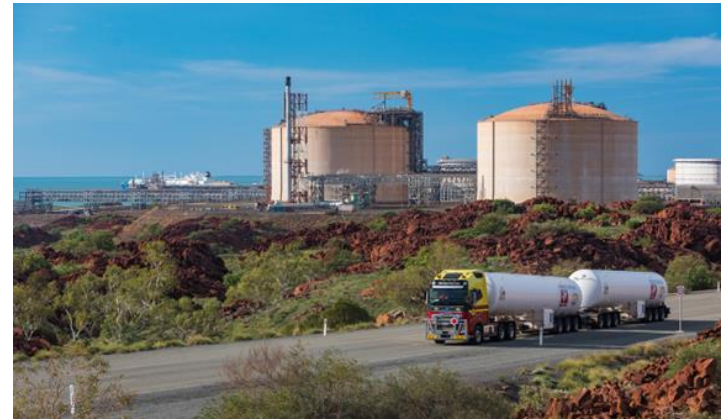
Image: LNG delivery via road train (Woodside's Pluto LNG Park and truck loading facility near Karratha in WA)
