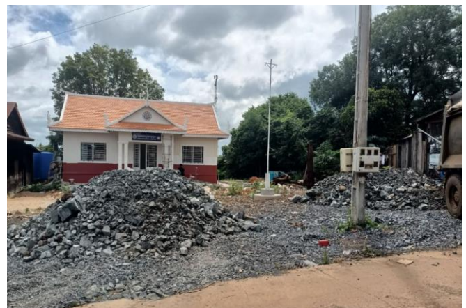
Figure 32 | Delivery of NAF waste rock to Chong Plah Police Station for driveway construction (2/2)
