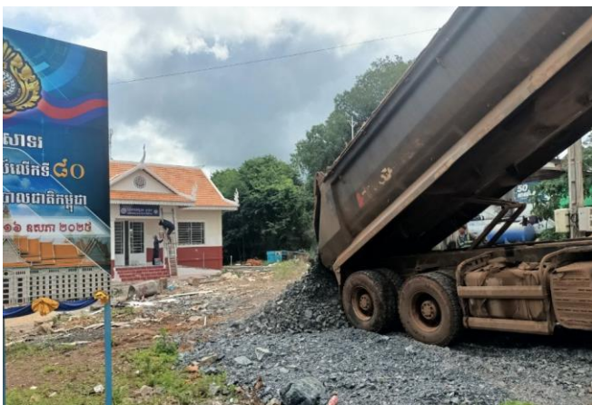
Figure 31 | Delivery of NAF waste rock to Chong Plah Police Station for driveway construction (1/2)
