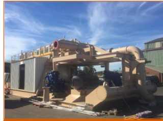
DMU Pump Skid Fabrication
