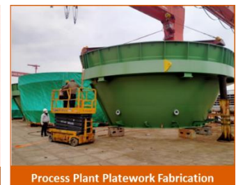
Process Plant Platework Fabrication
