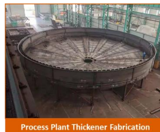
Process Plant Thickener Fabrication
