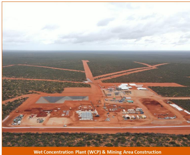
Wet Concentration Plant (WCP) & Mining Area Construction
