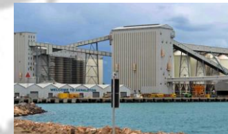
Coburn project DFS & funding phase
