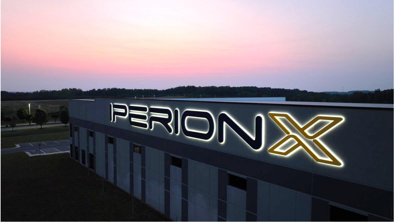
Figure 1: IperionX titanium metal production facilities at the Southern Virginia Technology Park in Halifax County, Virginia.
