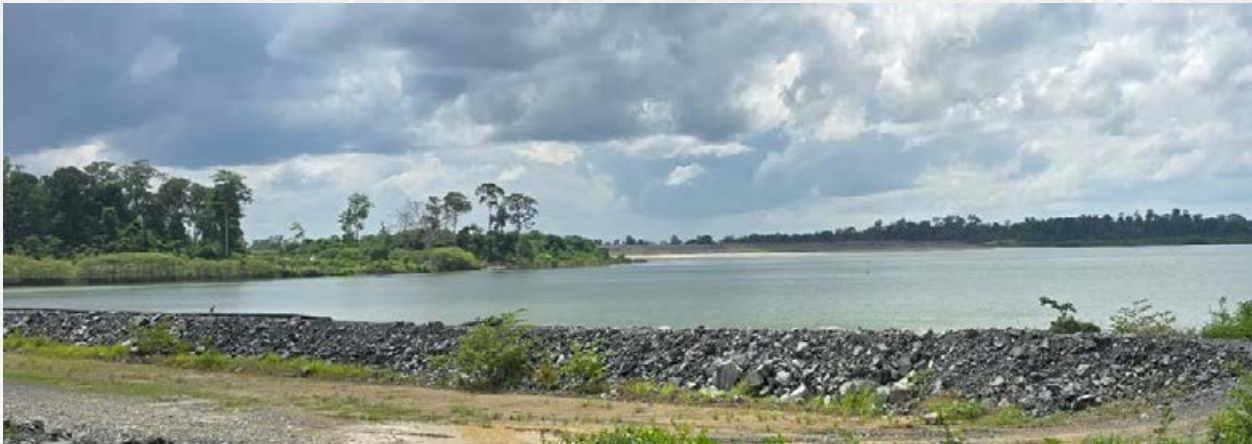
Figure 38 | Tailings Storage Facility at Okvau
