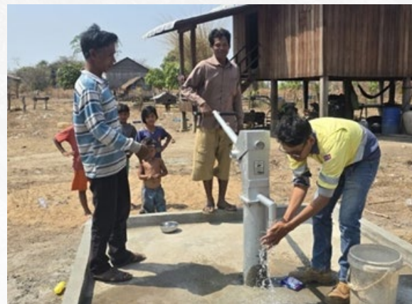
Figure 39 | Community water bore
