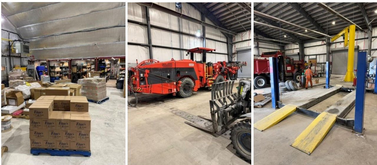
Figure 4: New indoor and insulated stores and workshops
