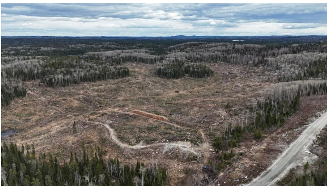
Figure 6: Tree clearing for the STMF completed
