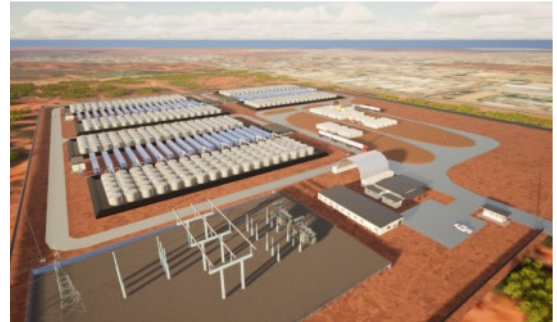
Rendering of AVL's proposal for a 50MW/500MWh VFB BESS in Kalgoorlie.
