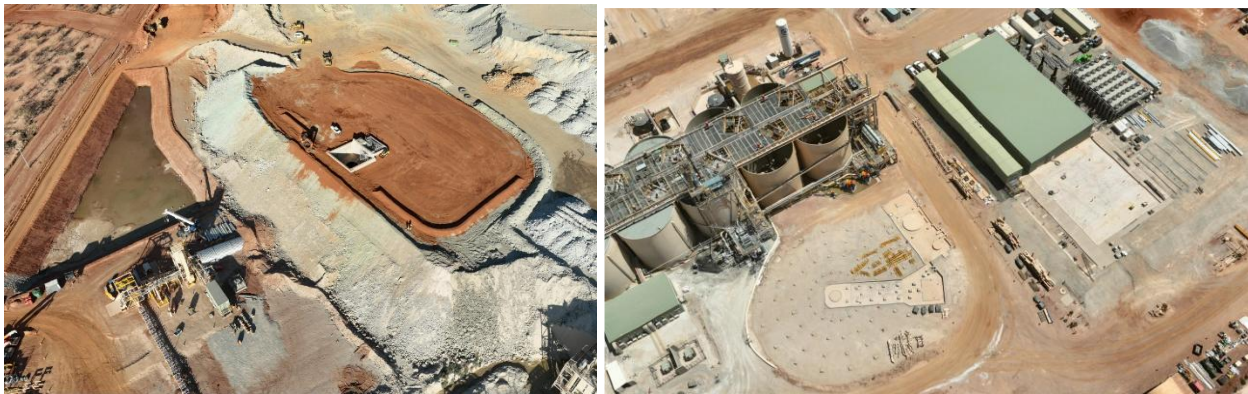
Figure 7: KoTH plant upgrade project - Primary crusher installation (LHS) and new CIL tanks, thickener and powerhouse extension (RHS)
