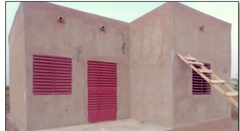
Dassa Clinic nurses' accommodation – Construction underway by Arrow Minerals
