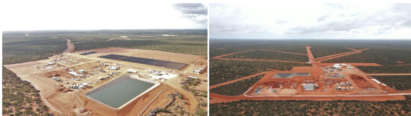
Figure 1 Coburn Project has reached 65% Complete and is On-schedule for First Production of HMC in December quarter 2022
