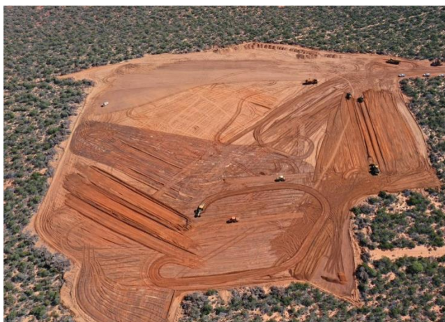
Figure 3 Village Bulk Earthworks Pad
