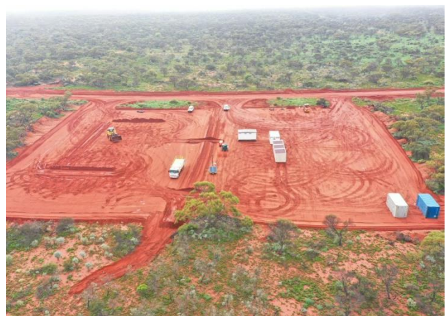
Figure 2 Preparing Construction Laydown Area
