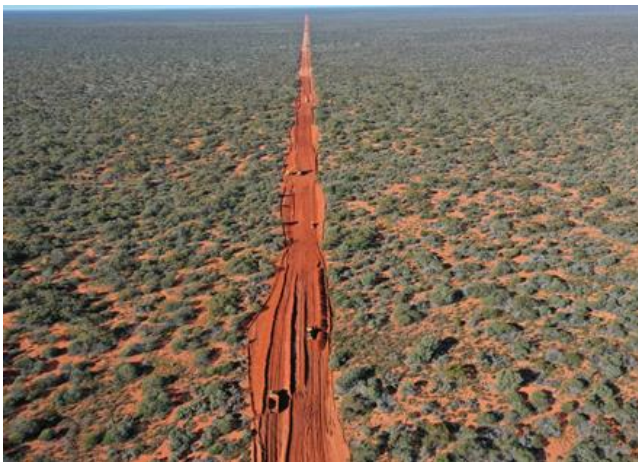
Figure 1 Construction of Main Access Road
