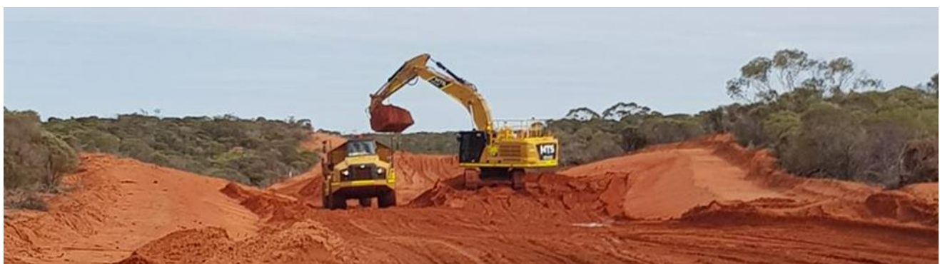
Figure 5 Construction of the Main Access Road
