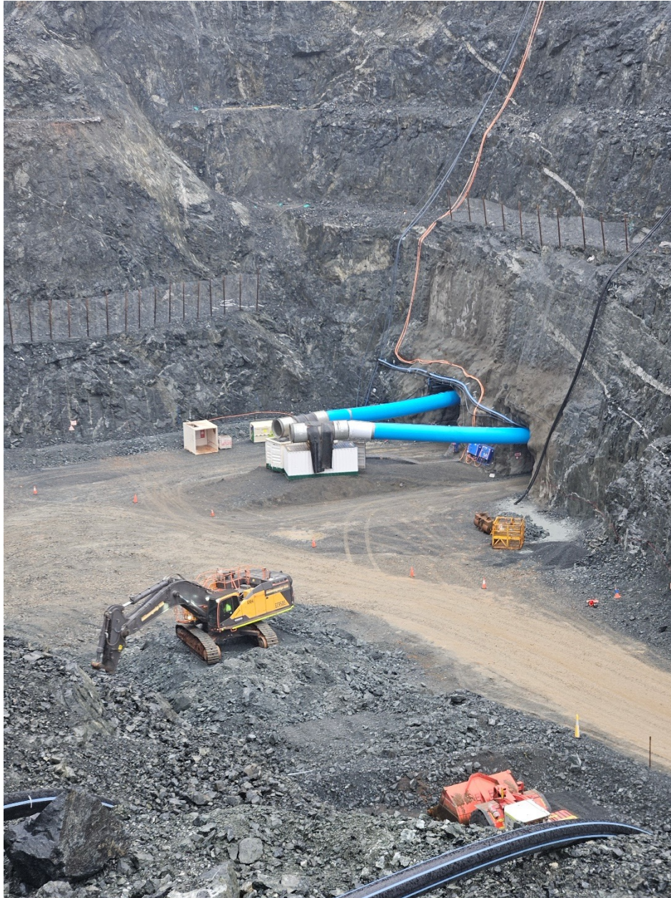
Figure 7 – Scotia portal and ventilation drive progressing ahead of plan
