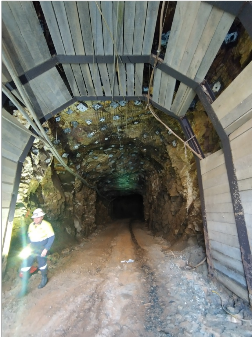
Figure 5 – Photograph from Bullen portal and decline development June 2024
